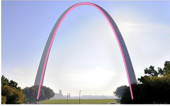
Figure 14. Structural expressionism form of the memorial arch resulted in inverting catenary in Saint Louis Gateway Arch, Saint Louis, Missouri, USA, Eero Saarinen (Architect) and Hannskarl Bandel (structural engineer), 1965 and hyperbola form on it. (Source of image: interestingamerica.com)
