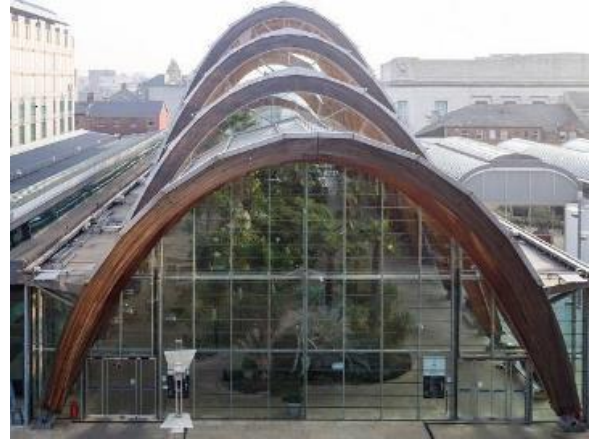
Figure 12. Glue-laminated two-hinged parabolic arches in winter garden, Sheffield, UK, Pringle Richard Sharrat Architects, 2002. (Source of images: prsarchitects.com and sheffieldnewsroom.co.uk )
