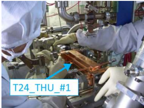
FIG. 3. Installation of the structure.
