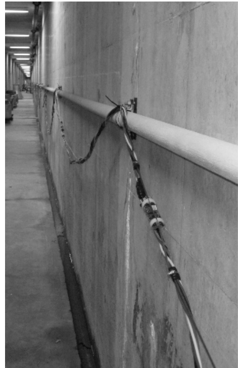
Fig. 7. Riser Modules Hanging in Corridor
