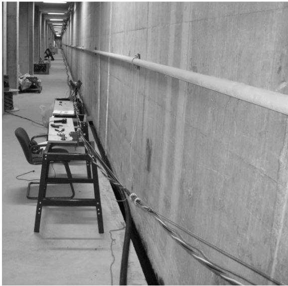
Fig. 8. Assembly Table and String of Modules
