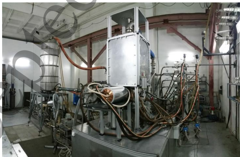
Figure 17. Shielded gyrotron system with HE 11 -mode waveguide, calorimetric millimeter-wave load and cooling water manifolds (gyrotron collector and load flow rates are 20 l/s and 10 l/s, respectively).
