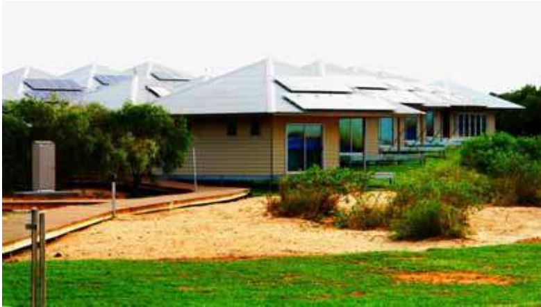
Fig. 18. Eco resort villas with photovoltaic panel installation
