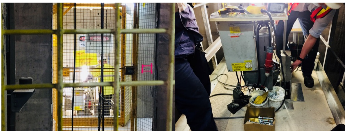
Figures 6.5 and 6.6: Assembling the “jump lift” on the construction site of a residential high-rise tower, Melbourne CBD, October 2017. Photo: L. Dorignon.
