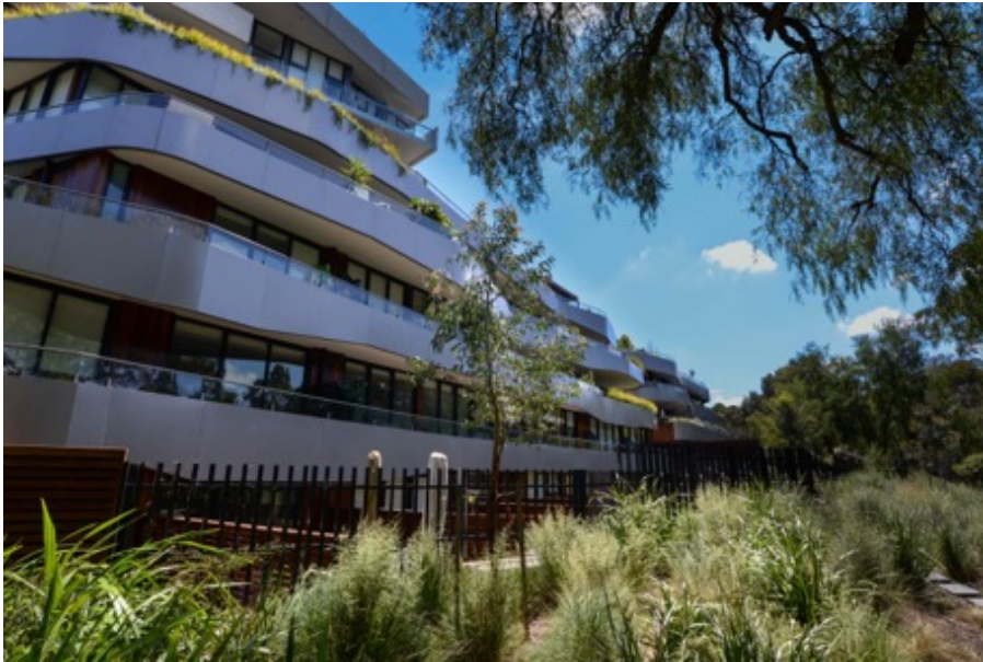
Figure 7.20: “A prime location”, view onto Haven’s balconies and terraces from the Yarra river path, October 2017. Photo: L. Dorignon
