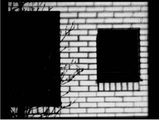
Fig. 15 Detection of the bricks in a small section of the scene above using SAM is shown. The variation in contrast with respect to the brick interval is due to aliasing.
