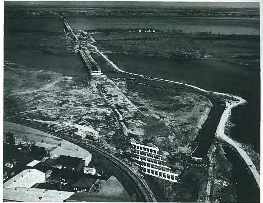
Fig. 28. An overview of the Champlain Bridge over the St. Lawrence and the Seaway at Montreal (built 1959-1962).
