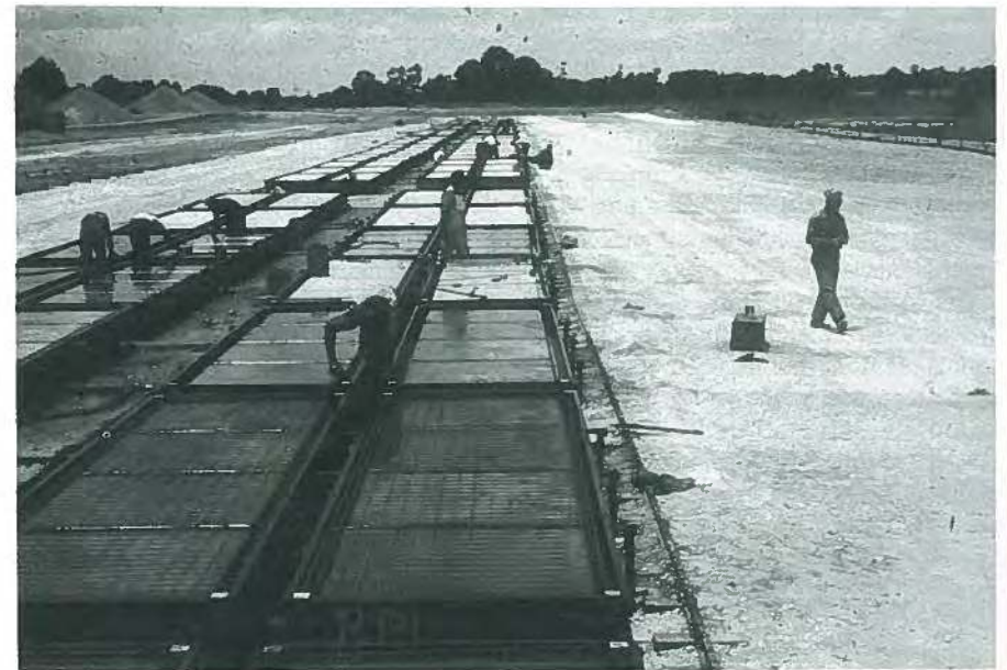
Fig. 26. Precast concrete installation at the U.S. Marine Corps Supply Depot in Albany, Georgia, 1952. One hundred and forty concrete molds permitted a daily production of 140 thin shell ribbed roof panels required for the 10 warehouses shown in the section above (Fig. 25).
