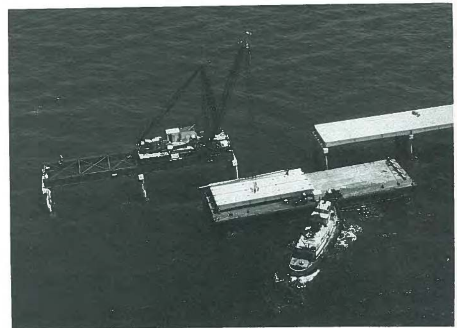
Fig. 7. General view of erection of a span to be part of the Chesapeake Bridge-Tunnel Crossing connecting Cape Charles to Norfolk, Virginia.
