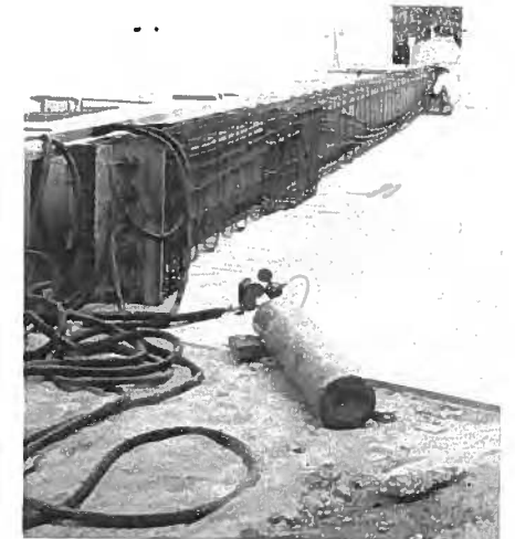
Fig. 19. Forms with inflatable rubber voids.
