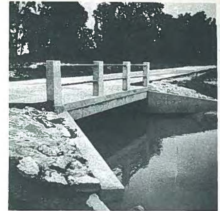
Fig. 14. Application of 14-in. (356 mm) double-tee for short-span farm-to-market bridge. Several hundreds of these bridges have been in use for over 20 years with excellent performance.
