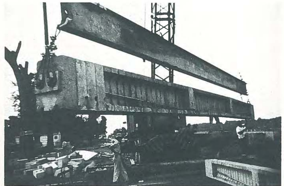
Fig. 16b (bottom). Close-up of block-beam during erection showing post-tensioning wire unit.
