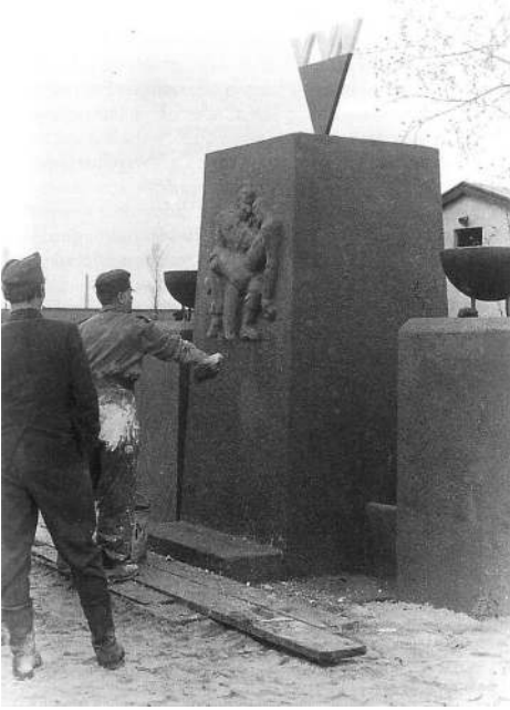
FIGURE 21: Provisional memorial in Sachsenhausen, 1954. This memorial, ca. 2.7 meters tall, was built from bricks from the camp prison, which had been demolished by state authorities against the wishes of the survivors. Photo from the Stiftung Brandenburgische Gedenkstätten/Archiv Sachsenhausen.
