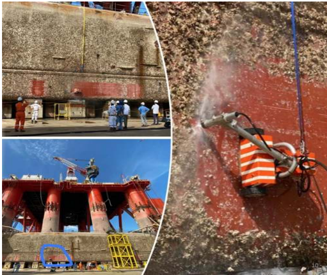
Figure 1: ShipHull surface with corrosion and blasting by Hornbil
