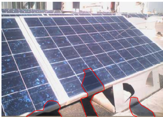
Figure 1: A multi-c-Si PV module which is shaded (red outline) from building services engineering.
