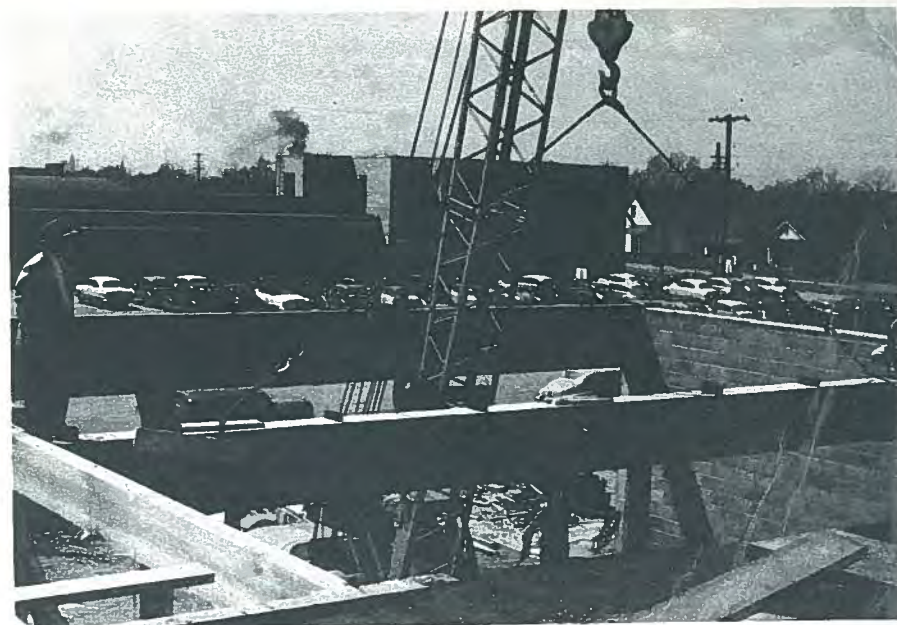
Fig. 14. The largest prestressed beam in Colorado made by Prestressed Concrete of Colorado was for the Plat Packing Plant in 1952.
