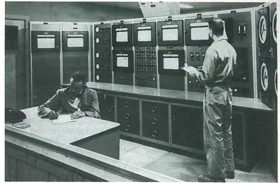
Fig. 38. Operating console in PCA's fire test center.
