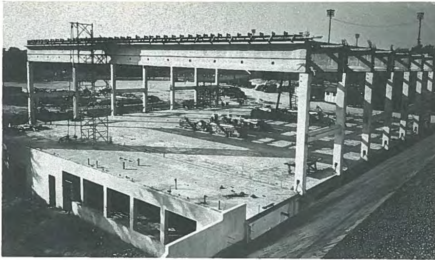
Fig. 41. All prestressed girders in place for Greensboro, North Carolina, Senior High School gymnasium.
