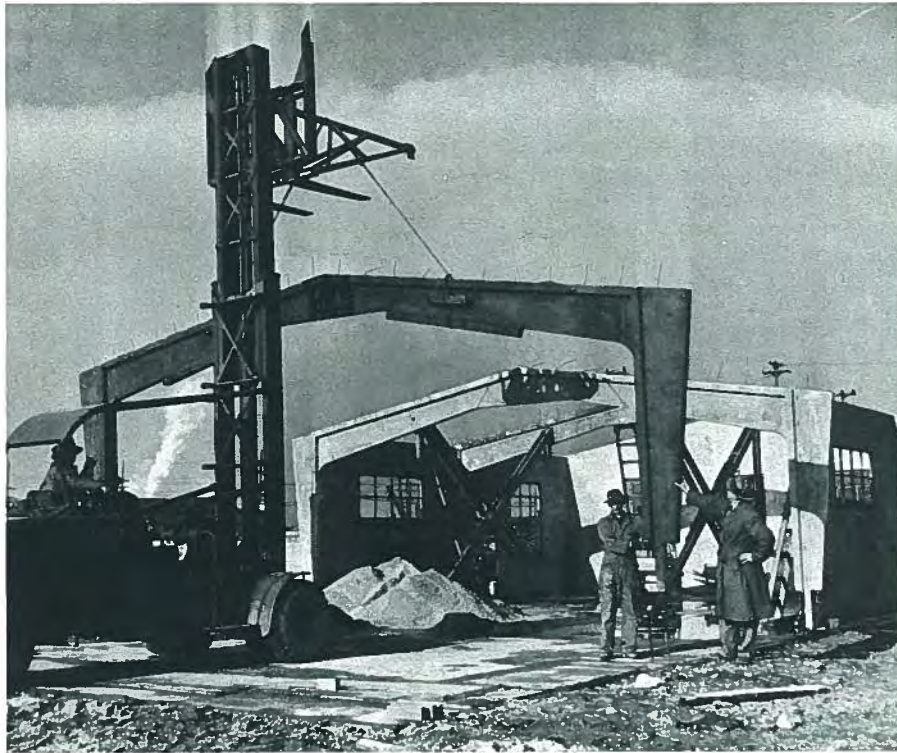
Fig. 43. Erection of Concrete Engineering Company shop building (1951).
