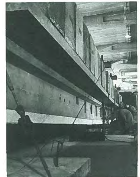
Fig. 69. Load test of beam with nine web openings for Norton Building at Concrete Technology pilot plant.
