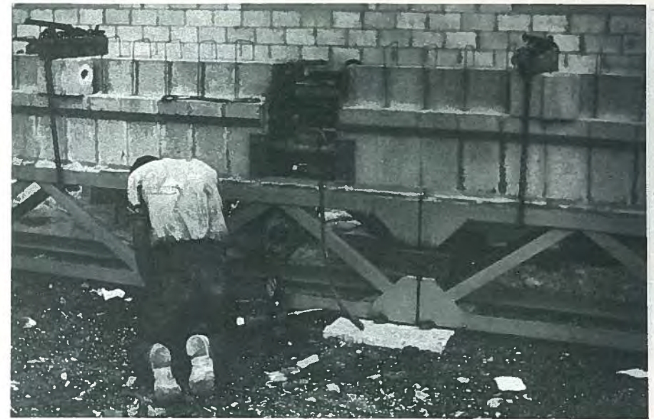
Fig. 10. Tensioning two 16x24-in. (406 x 610 mm) block building beams by jacking them apart.
