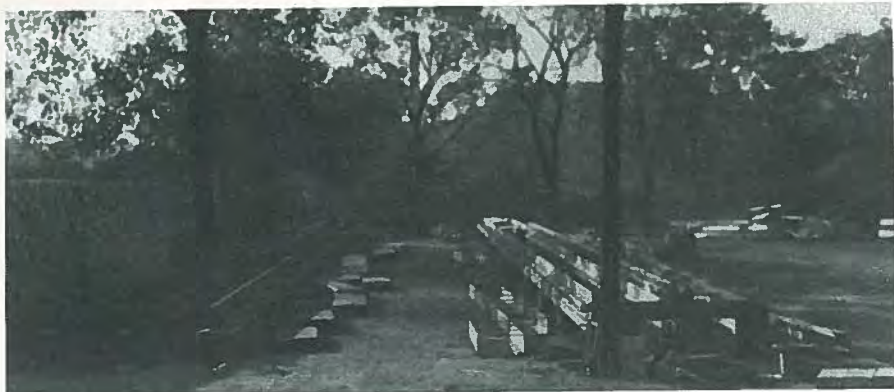
Fig. 16. Fabricating beds at a Breeko plant for producing pretensioned channel slabs with deflected strands. Built in March 1953.
