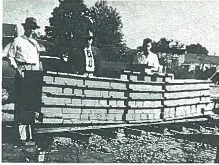
Fig. 30. Testing of soffit beam made up by masonry blocks (Tulsa, Oklahoma).
