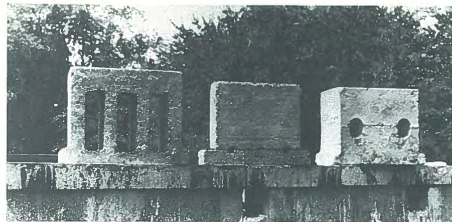
Fig. 4. Madison County Bridge beam units.
