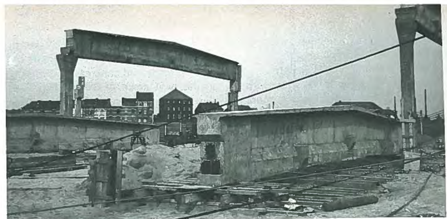
Fig. 34. Prestressing wires locked in position at end of beam.
