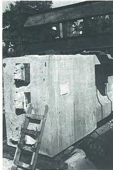
Fig. 8. West end of Walnut Lane test girder, showing clinometer. Strain gage load cell is located over jack.
