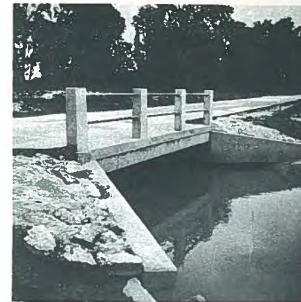
Fig. 14. Application of 14-in. (356 mm) double-tee for short-span farm-to-market bridge. Several hundreds of these bridges have been in use for over 20 years with excellent performance.
