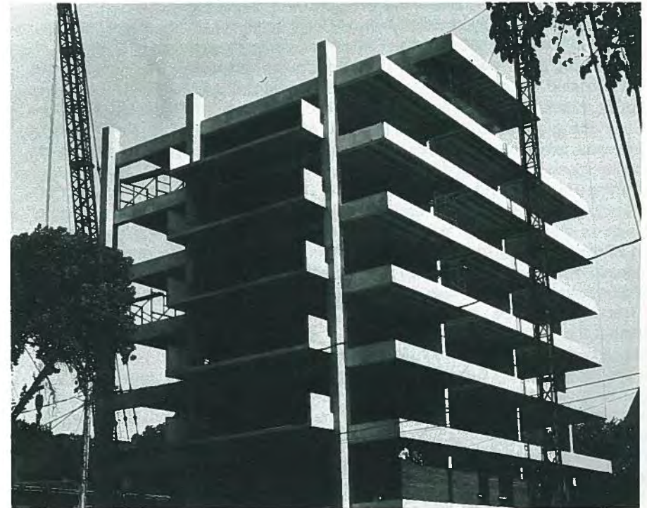
Fig. 24. Grosvenor House in Winnipeg, tallest all-precast building in Canada at the time of its construction (1960).
