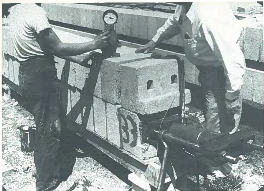
Fig. 2. Tensioning stadium beams.
