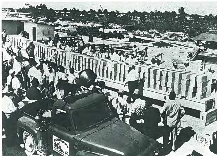
Fig. 25. Demonstration test of 100-ft (30.5 m) long prestressed channel slab at R. H. Wright & Son, Fort Lauderdale, Florida.
