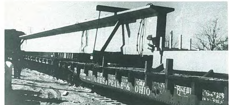
Fig. 22. Milan Gymnasium girders, 102 ft (31.1 m) long, with deflected strands. Built in 1955.
