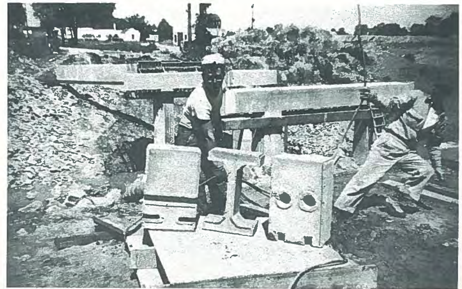
Fig. 12. Typical Michigan area blocks as produced by Besser machine.
