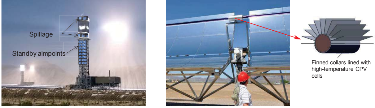
FIGURE 1. Conceptual design of PV cells on heat shields or standby regions of a central receiver (left) or on the bellows shields of a trough receiver (right).
