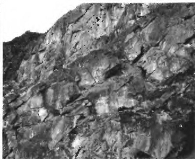
FIGURE 5. — Secondary openings along bedding and joint planes in Cambrian(?) carbonate rocks, Titus Canyon, Death Valley National Monument, Calif. Openings in middle ground, up to 10 feet long.
