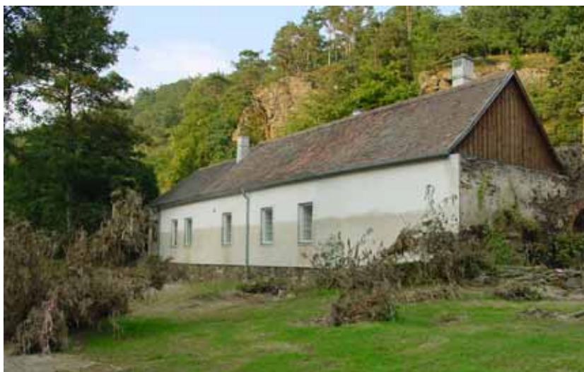
Fig. 2 Flood marks of the August 2002 flood at the bank of the Kamp near Rosenberg (Reach 5). The peak flow was about 570 m 3 /s. Photo courtesy of Pfarre Horn.
