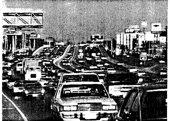
Exclusive HOV Facility in Freeway Right-of-Way, Houston, Texas, Katy Freeway
