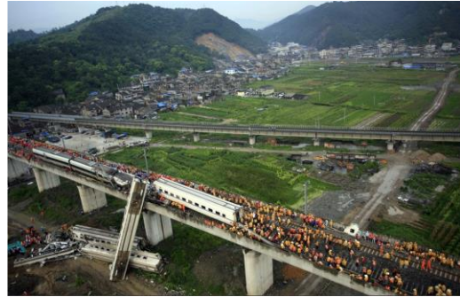
Figure 7. Derailment accident happened in Wenzhou, China
