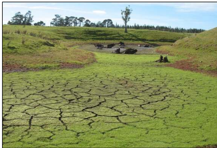
Figure 4.16: Cracking was observed in the dry sections of all three ponds during the summer and autumn study period. Photo shows cracking in Pond C, looking downstream towards the remaining stored water.
