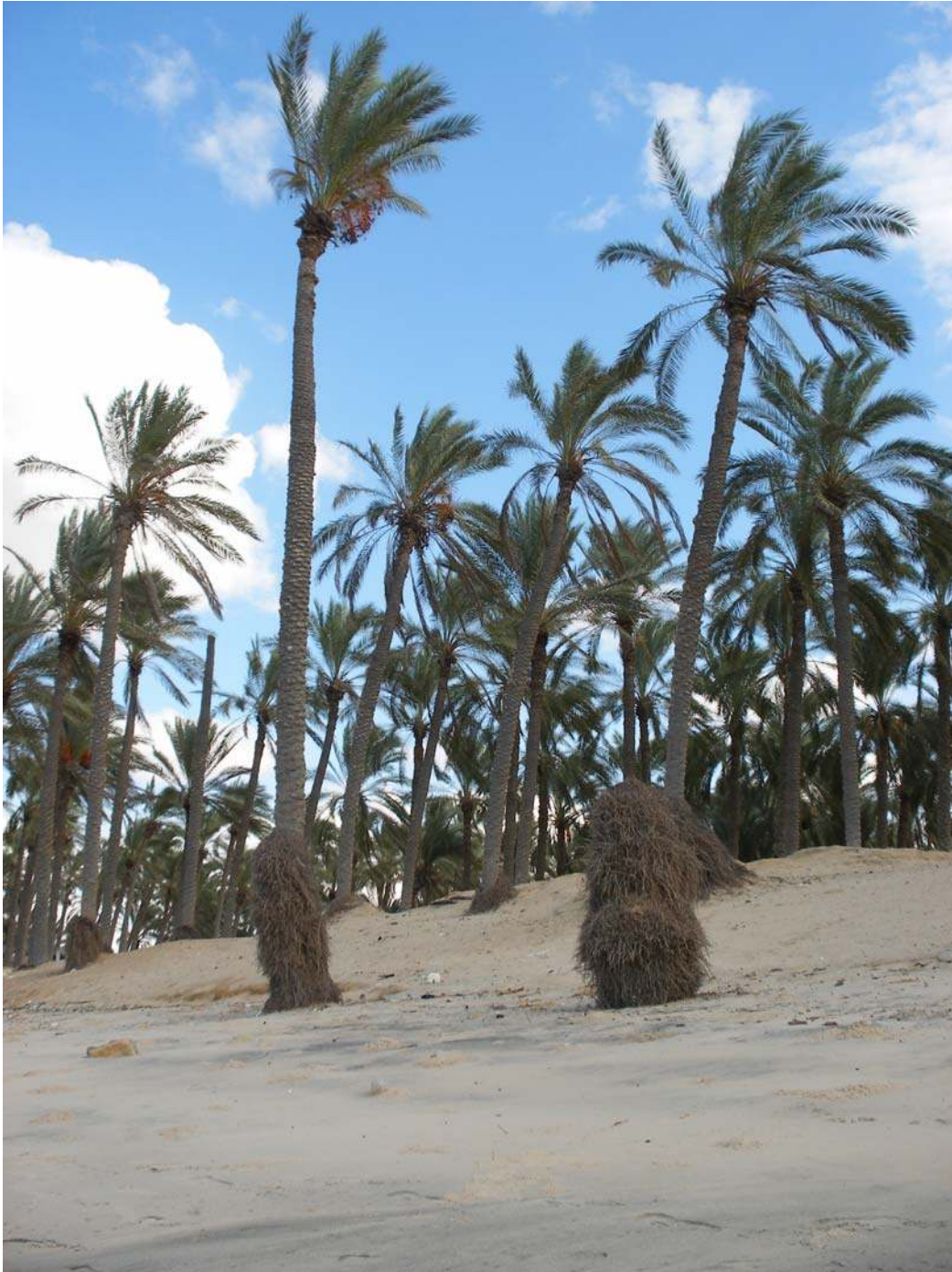
Figure 1.1 Exposed roots of palm trees indicating severe erosion along the beach in the east of El Arish Harbor.
