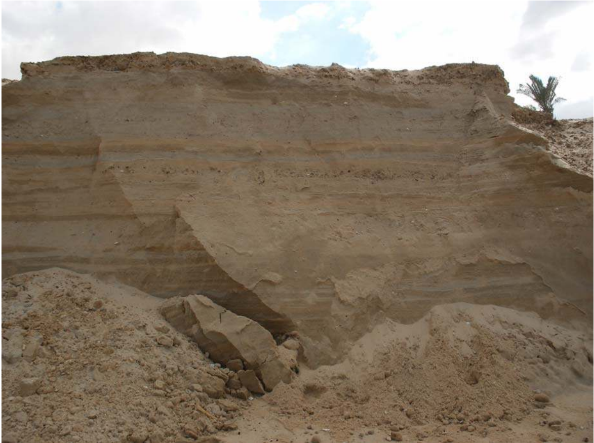
Figure 1.2 Erosion of sand dune at the palm beach east of El Arish Harbor.
