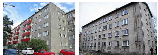
Fig. 1. Typical prefabricated reinforced concrete large-panel element apartment building (left) and brick apartment building (right)
