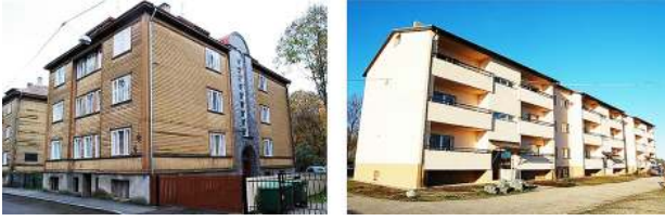
Fig. 2. Typical wooden apartment building (left) and autoclaved aerated concrete large-block building (right)
