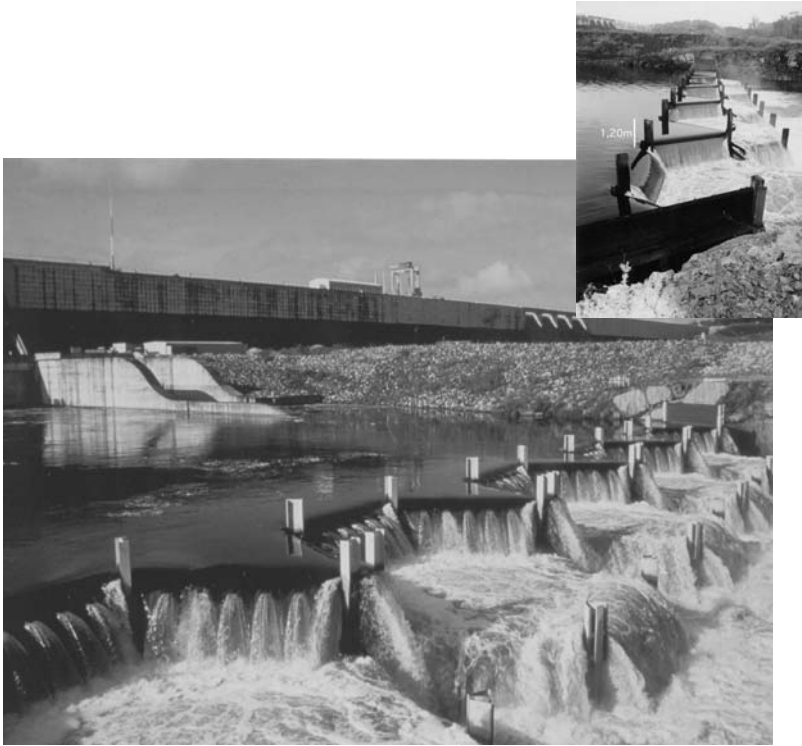
Fig. 22.9. Aerating weir in the power plant outlet canal before and after its first lowering
