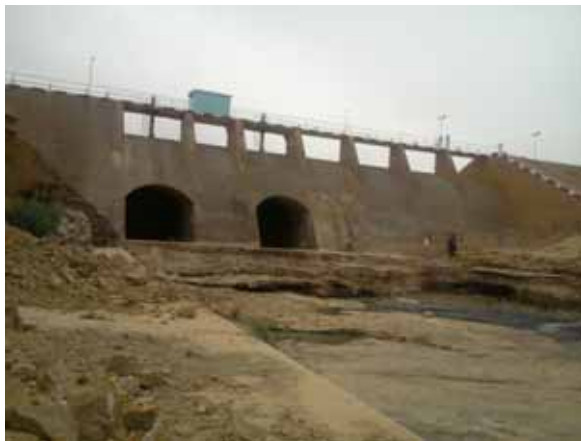
Fig. 3. An overview of the Boughezoul dam; photo: B. Remini
