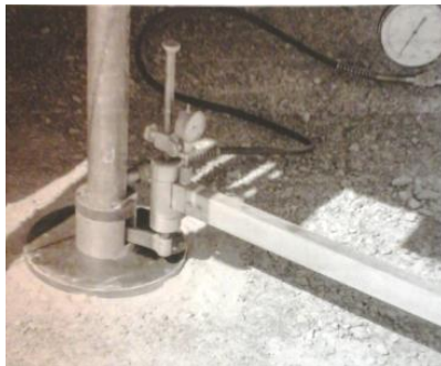
Fig. 3. General view of the loading plate for static tests.
