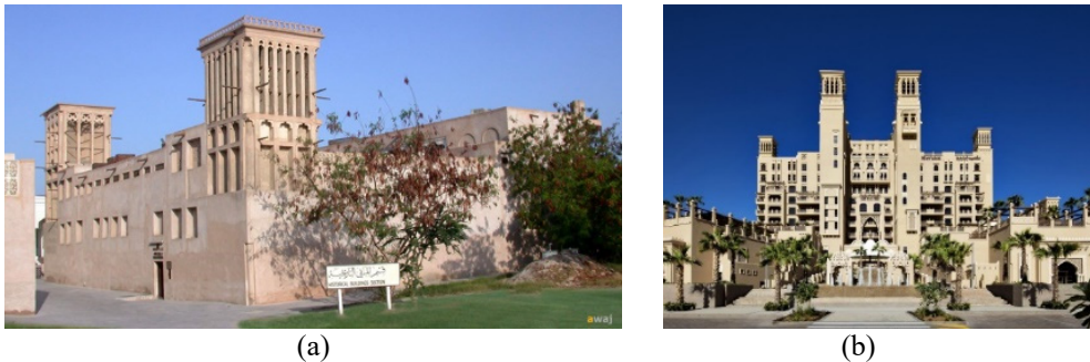
Figure 2: (a) A traditional house in a Fahidi District (Dubai) where it uses a wind tower (called Barajil ); and (b) The Sheraton Hotel in Sharjah, where the Barajeels are just part of the décor. (Source: The authors. )
