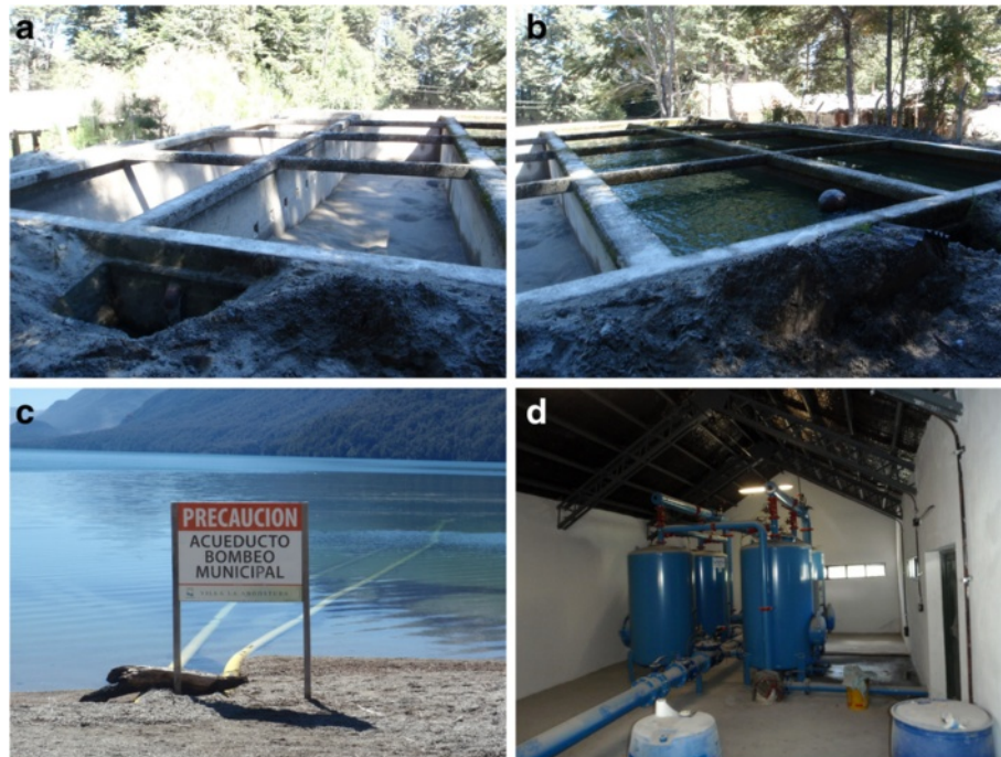
Fig. 8 Villa la Angostura water supplies a non-operational sand filters of the Las Piedritas stream-fed system, filled with ashfall; b operational sand filters at the Las Piedritas treatment site; c Lomas del Correntoso intake from Lake Correntoso; d Chlorination plant
