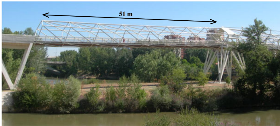
Figure 2. View of span 2.
