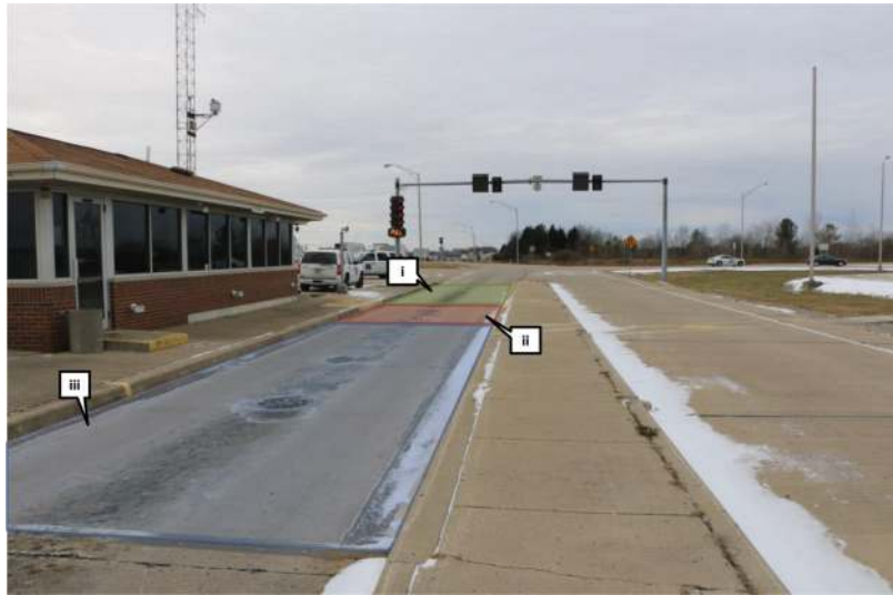
Figure 4.7 Indiana State Police weigh scale at Richmond.
