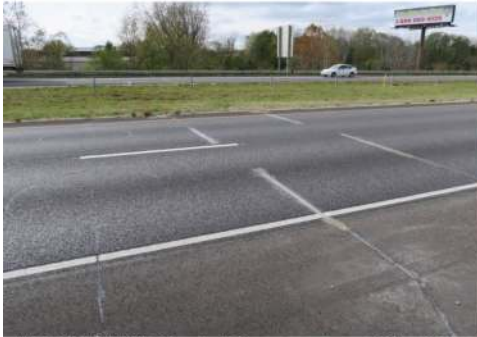
(b) WIM #3700 Physical Components and Condition
