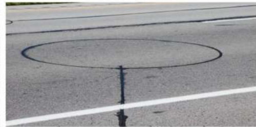
(c) Inductance loop at WIM station
