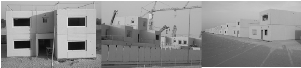
Figure 2: Erection of Villas
