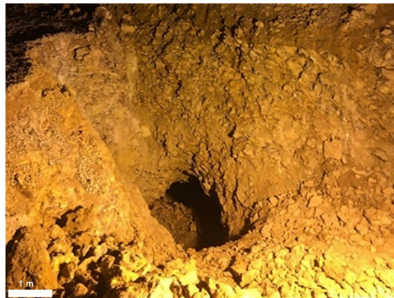
Fig. 7 Karst cave encountered during tunnel excavation in dolomitic limestones
