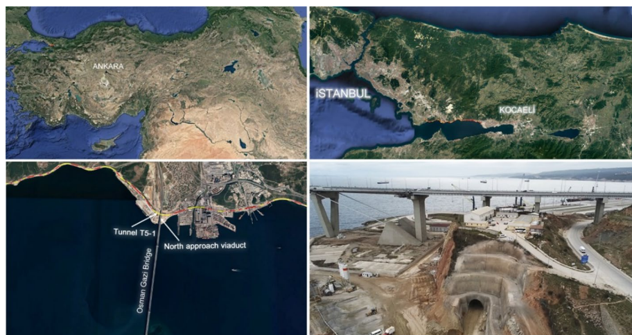
Fig. 1 Gebze-Köseköy project and T5-1 Tunnel location (Google Earth)
