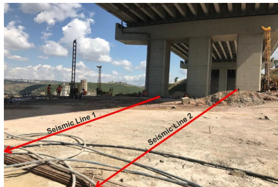
Fig. 12 Distribution of the MASW measurement point over the tunnel
