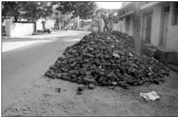
Construction and demolition waste is deposited onto a street.
