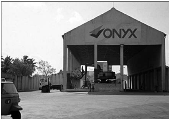
A transfer station is appropriate when the treatment and disposal site is far from the city.
