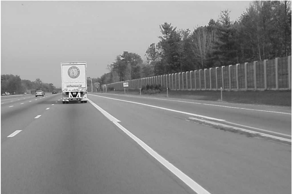
Figure 3 Noise barrier reducing noise entering residential community
