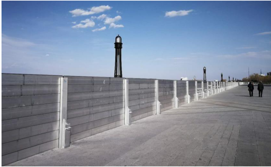
Figure 19. The view of the removable floodwall.
