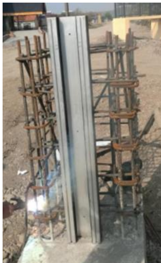
Figure 14. End post welded to the reinforcement.
