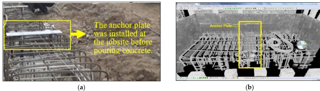
Figure 13. Anchor plate in the job site and point cloud. (a) Anchor plate in the job site and (b) anchor plate point cloud.
