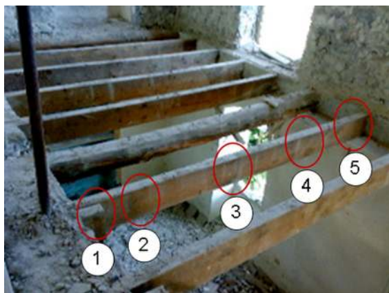
Fig. 5 Typical example for stress wave based condition assessment in structural timber
