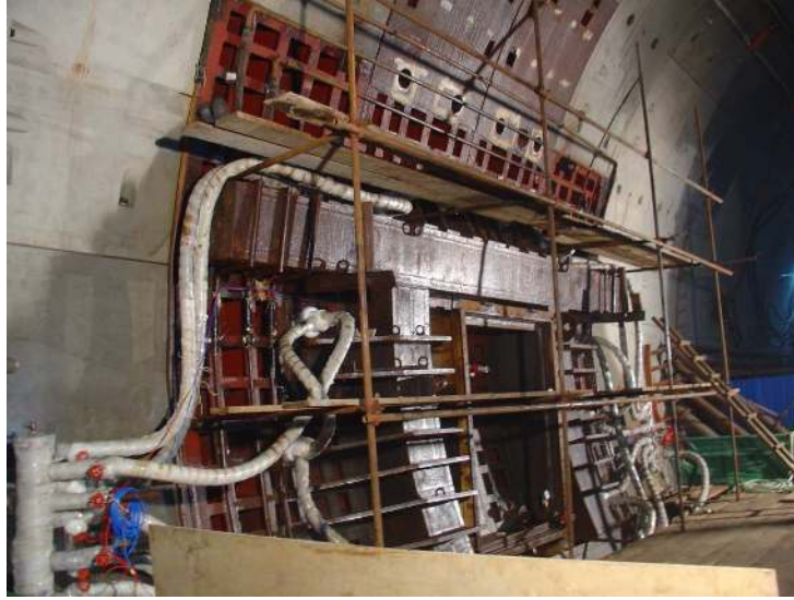
Photo 3. Photo taken in front of steel segments at the start of freezing
