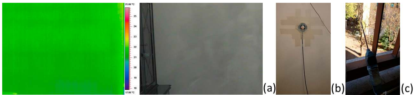
Figure 3. (a) Wall's thermographic investigation; (b,c) heat flow meter sensors.
