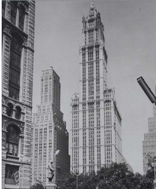
A view of the Woolworth Building, which housed Fordham University School of Law from 1915 until 1945.
