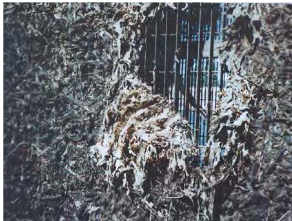
Figure 18. Stalks of D. geminata clog a grate in a water supply canal in California. (Image by Peter Pryfogle, Idaho National Laboratory.)
