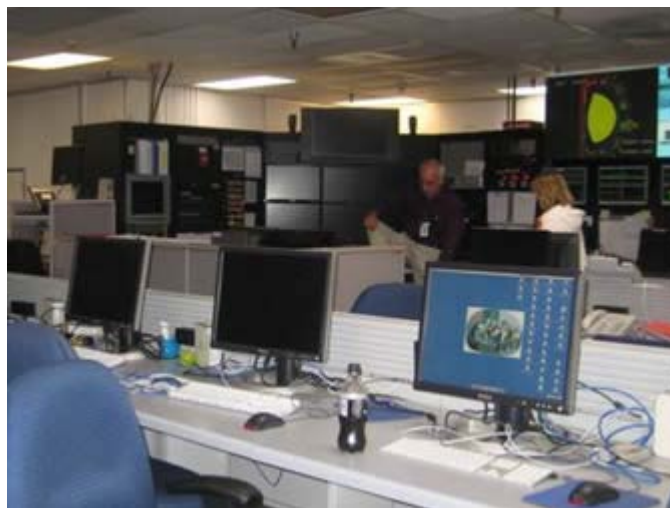
Figure 6. General Atomic control center room showing technology resources.
