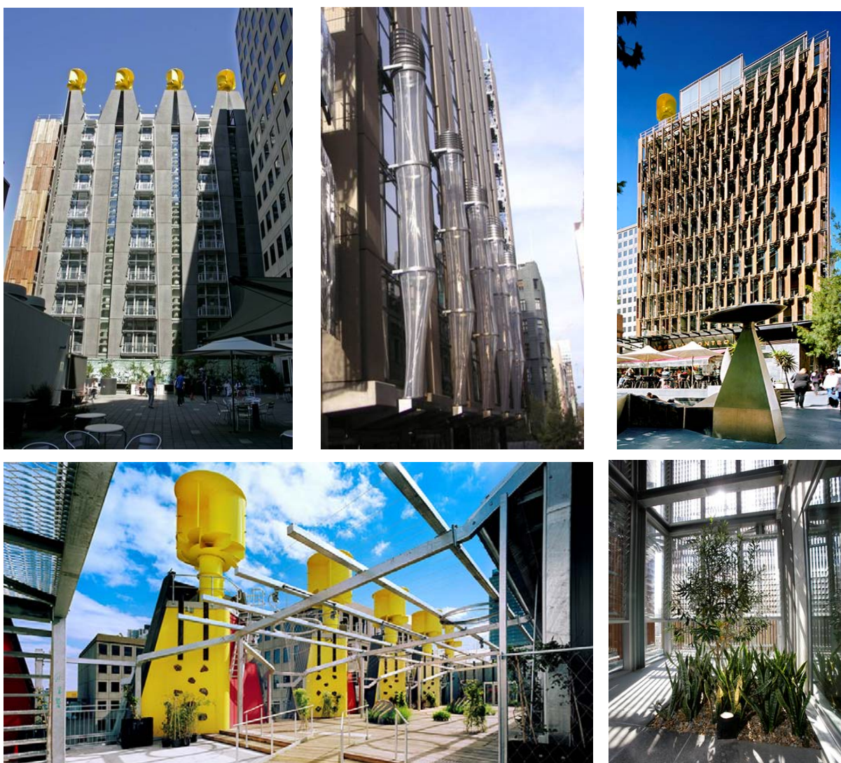
Figure 1: Exterior views of CH2
