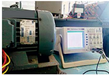
FIGURE 2: Experimental setup of 5 hp three-phase induction motor with interturn fault in one phase.
