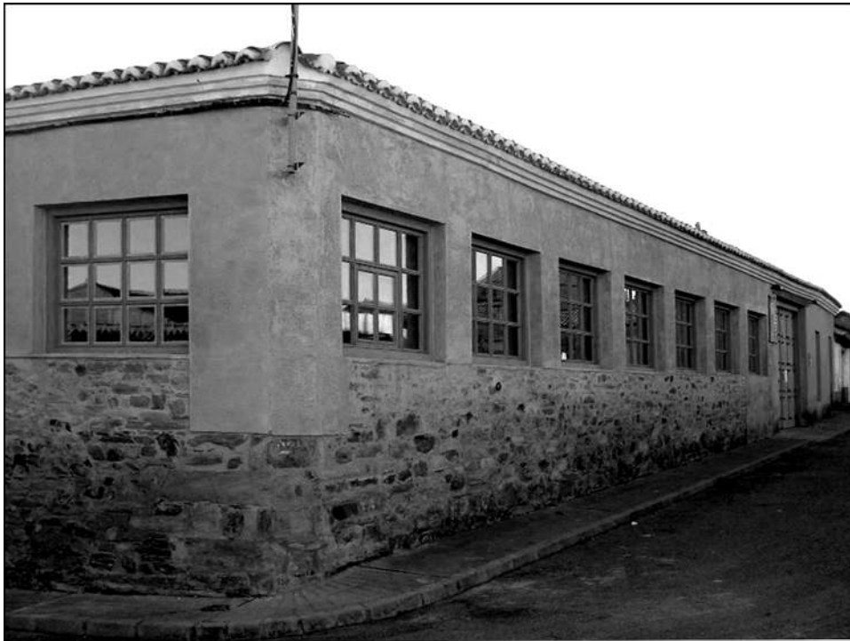
FIG. 4—The same former communal factory shown in Figure 3 after its conversion into an interpretive center. In hope of attracting tourists, the concrete was removed from the walls so the stones are now visible. Fresh paint and a new roof, windows, doors, and interior decor have rendered the building more like traditional-vernacular architectural standards in the area and less “industrial.” (Photograph by Pablo Alonso, November 2008)
