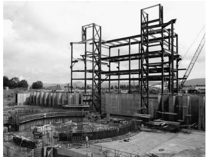
FIGURE 2. Looking north from Switchyard 1. (40-60-0598-1007#3pb02)
