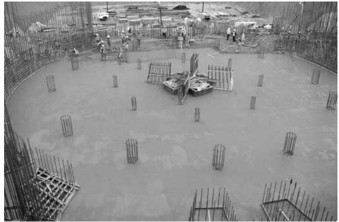
FIGURE 3. Finishing the Target Bay slab. (40-60-0398-0616#20pb01)
