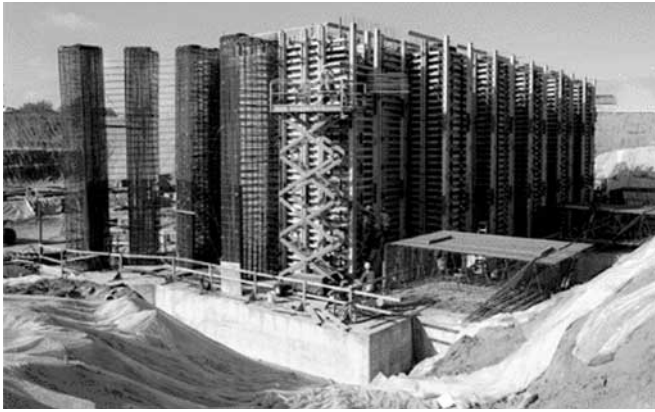
FIGURE 2. Target Area retaining wall forms and rebar. (40-60-0198-0084#46pb02)
