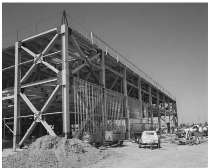
FIGURE 1. Installation of metal studs in the OAB. (40-60-0998-1855#11)
