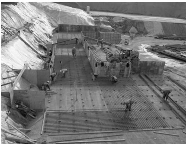
FIGURE 1. Target Bay footing construction. (40-60-1297-2604pb01)
