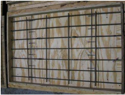
(a) Typical Formwork
