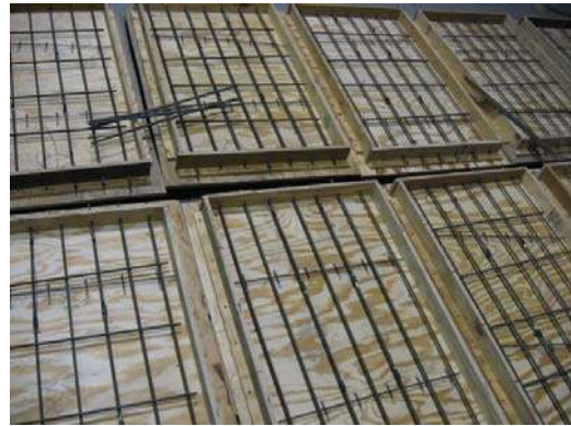
(b) Slab forms prior to casting
