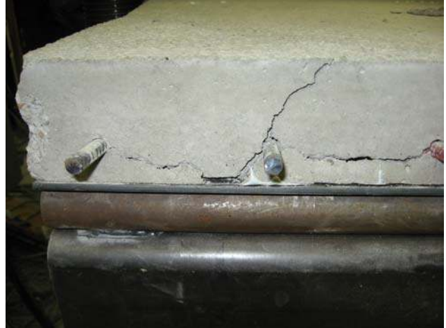
(d) crack at the level of reinforcing bars on the southern face of Specimen 12x1
