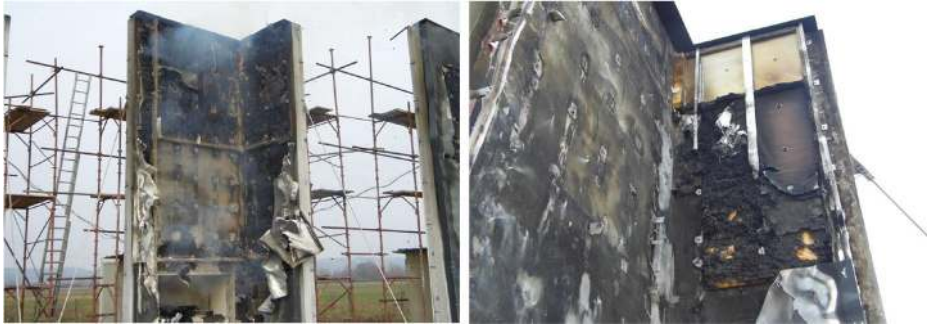
Figure 12. Sample 6 and 7- influence of vertical barrier on fire spread.
