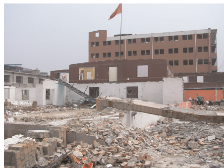
Figure 1. The demolition of Tangjialing.
