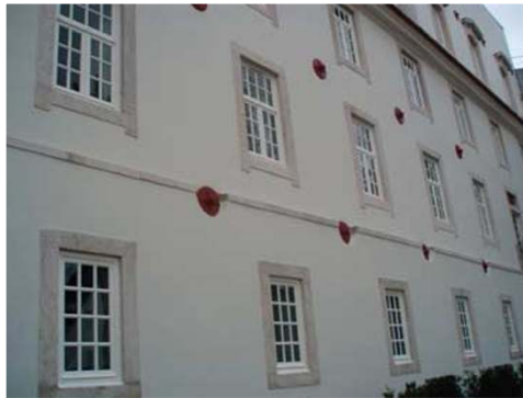
Figure 20: General view of the final appearance of the East Façade finishing.
