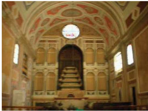
Figure 2: Church with lime plaster simulating marble.
