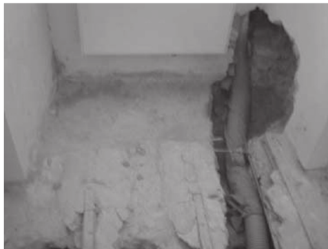
Figure 16: Introduction of the ventilation tube in the underground tunnels.
