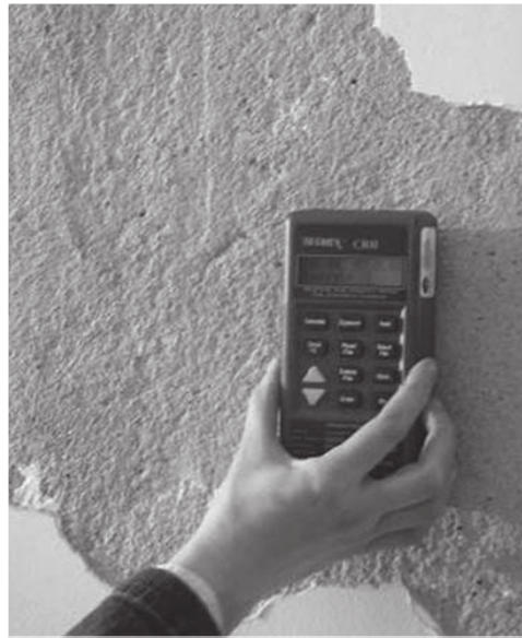
Figure 9: Evaluation of the moisture content with portable humidimeter.
