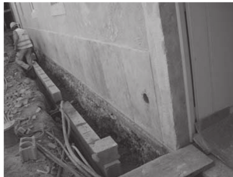
Figure 13: Execution of a ventilation ditch near the building façade.
