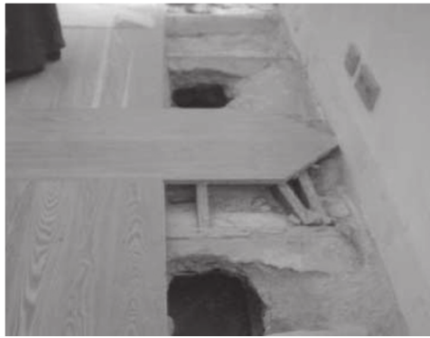
Figure 15: Small tunnels were opened under the ground floor.
