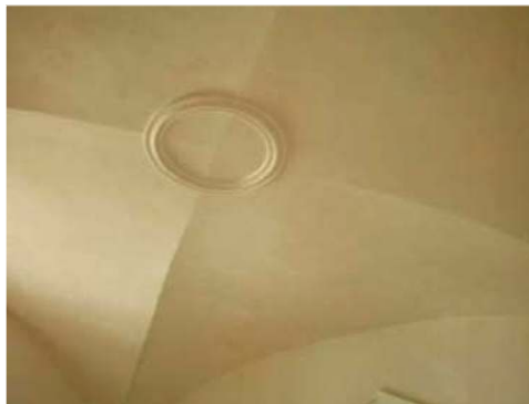
Figure 19: Application of traditional plaster on the ceiling of apartment 4.6.
