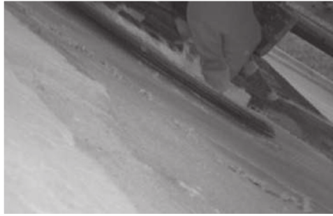
Figure 17: Application of the lime finishing coat.
