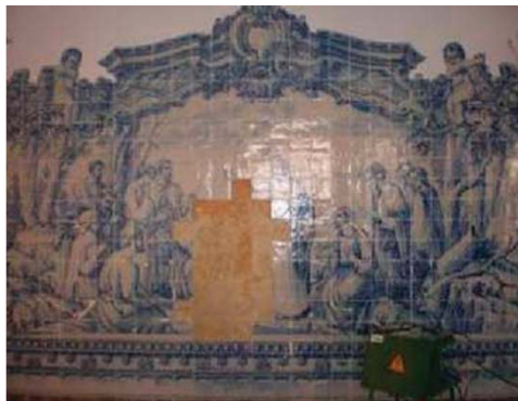
Figure 3: Lacuna in the interior glazed tiles ('azulejos') showing the old lime plaster.
