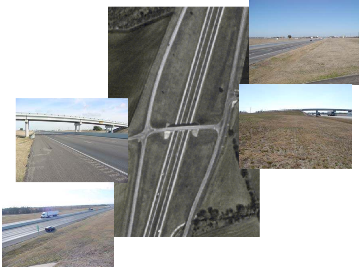
Figure 26. Site “D” Aerial Photo with Ground Photos Looking North and South from the NE and SW Quadrants.
