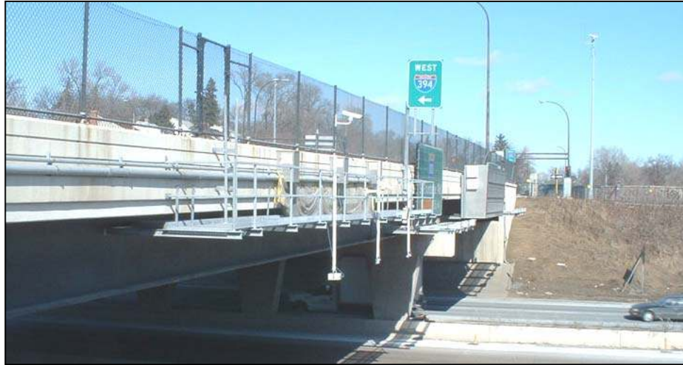
Figure 6. Catwalk for Mounting Detectors Overhead.
