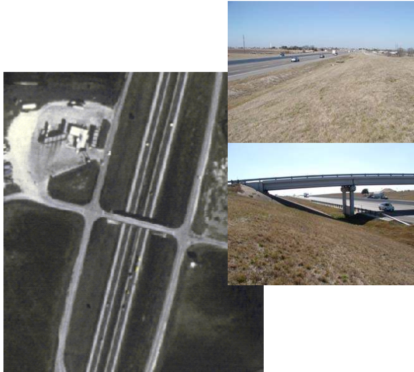
Figure 25. Site “C” Aerial Photo with Ground Photos Looking North and South from the NE Quadrant.
