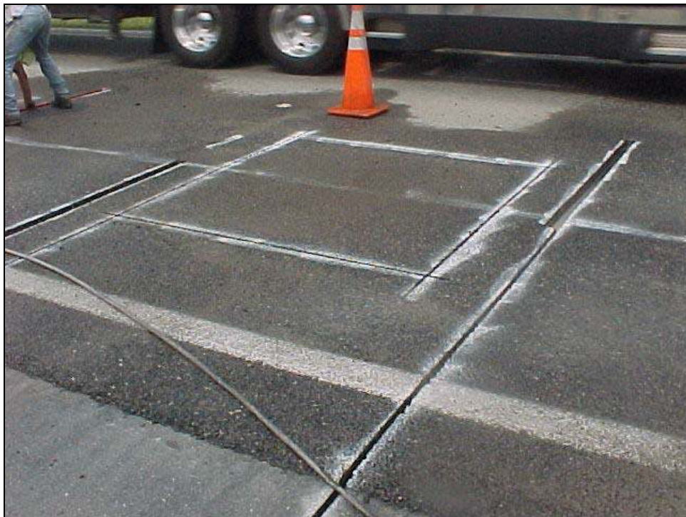
Figure 3. Kistler Sensor Saw Cuts During Installation.
