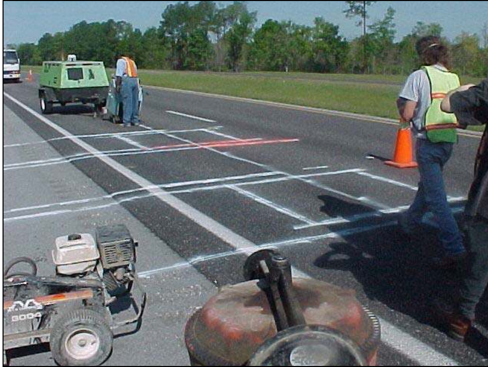
Figure 2. Kistler Sensor Layout Before Installation.
