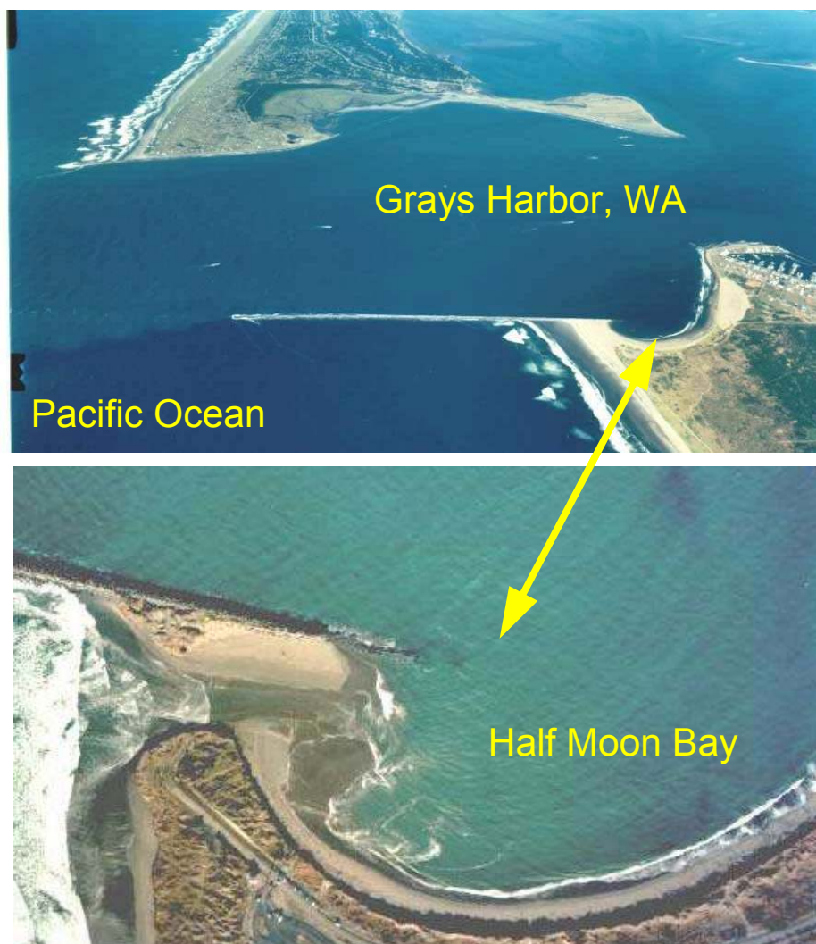
Figure 5. Jetty flanking at Half Moon Bay, Grays Harbor, WA
