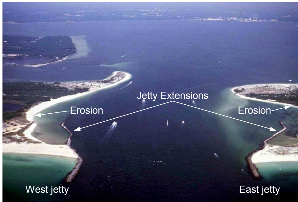
Figure 4. St. Andrews Bay Inlet (Panama City, FL) 1992. Jetty extensions added to prevent flanking
