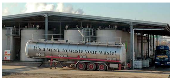
Fig. 3. Courtesy of De Neef Chemical Processing, Belgium
