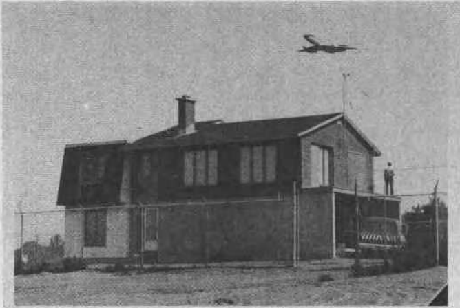
FIG. 1. Building constructed for experimental measurements, as viewed from the south.
